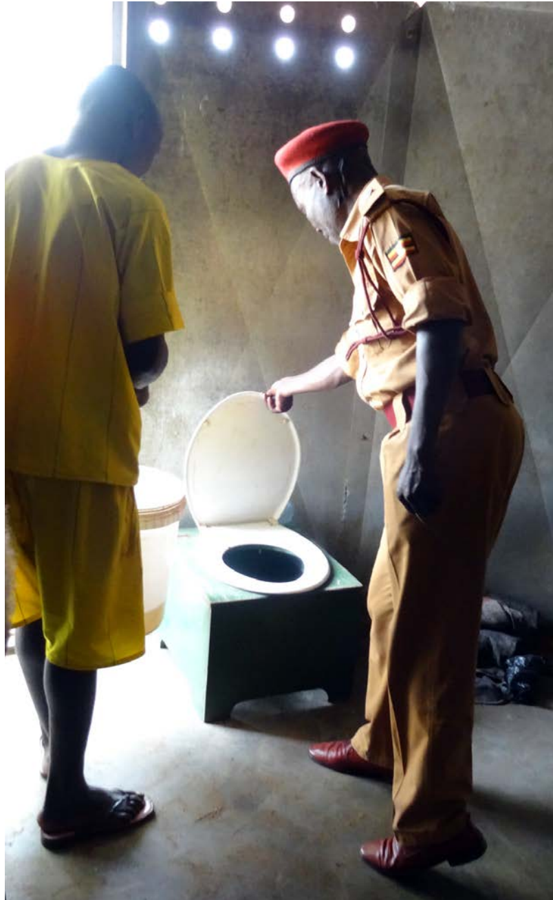
Figure 3-Patrick, the chief officer, shows off a compost toilet in the uniport at the Nakapiripirit prison.
