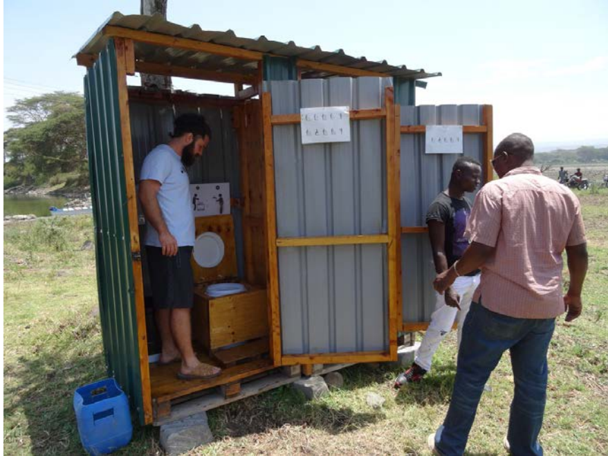
Figure 7-Compost toilets at Lake Naivasha, Kenya.
