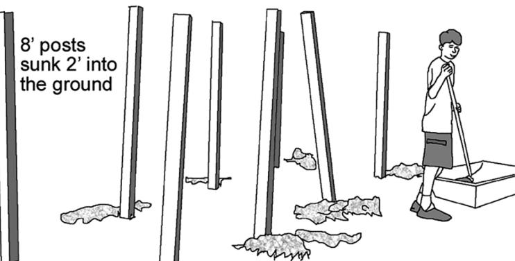
with concrete. Posts are about 5' (1.6 meters) apart. Leave four center posts high. Cut four outer posts to a height of about 4'.
